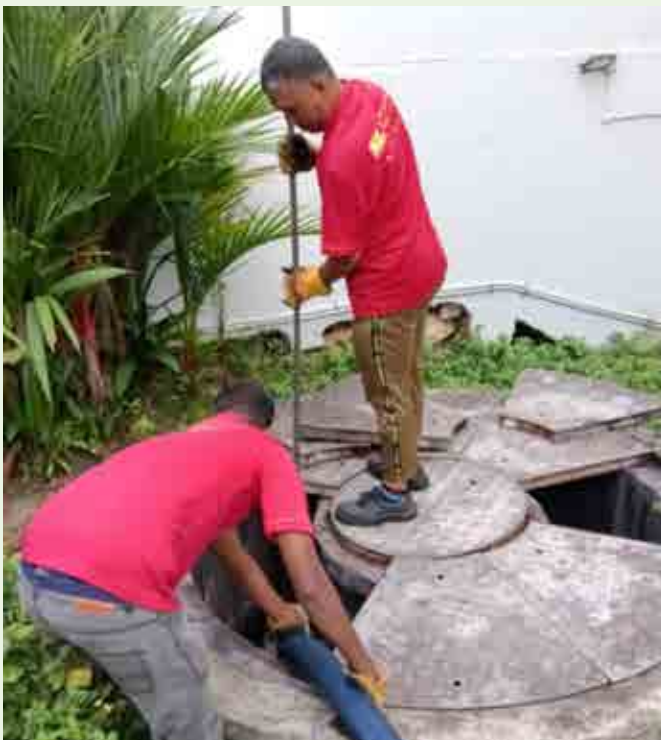
Contractors carrying out scheduled maintenance and cleaning of the grease interceptor system.
