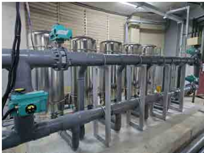
New energy-efficient filtration system installed to improve pool water quality and reduce operating costs.
