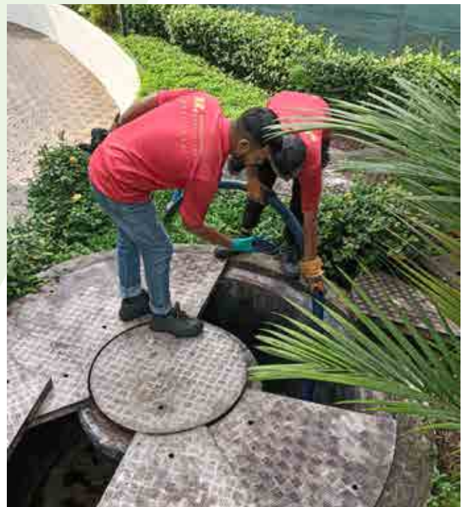
Contractors carrying out scheduled maintenance and cleaning of the grease interceptor system.
