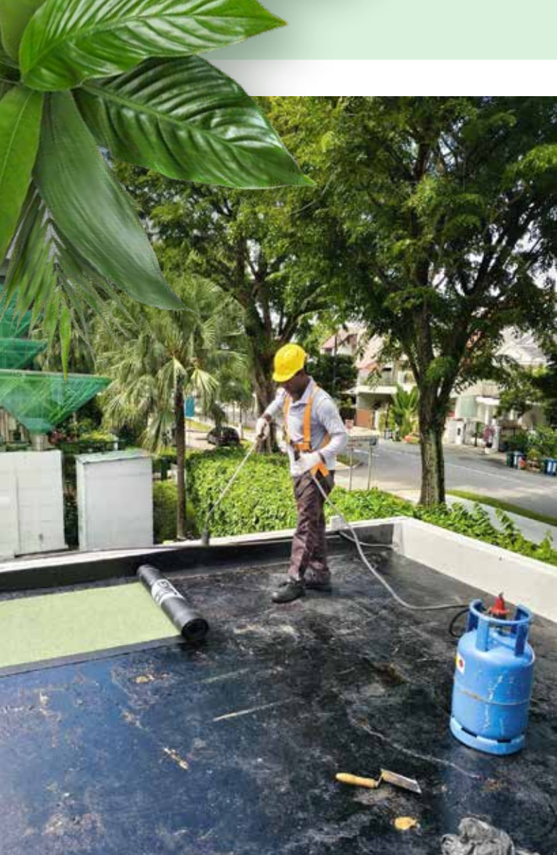
Above: Waterproofing works carried out at the substation area.
