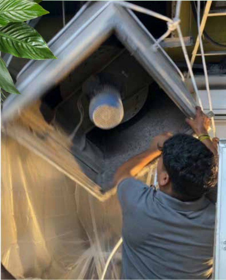
Above: Replacement of the ageing kitchen exhaust motor.
