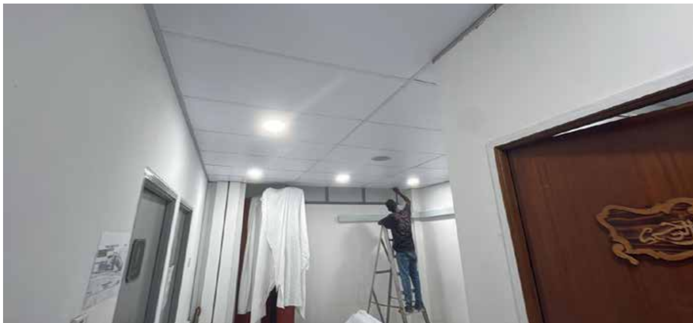
Above: Upgrading works for the staff lounge and rest room.
