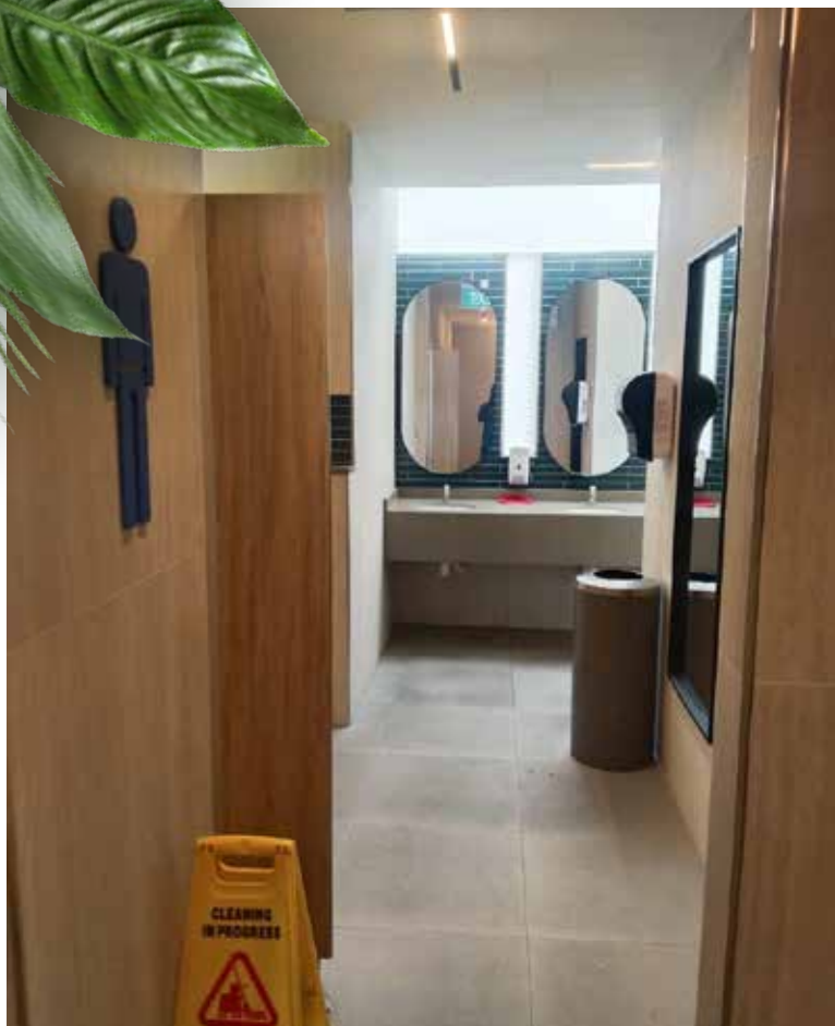
Above: Renovated atrium toilets with upgraded fittings.
