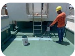
5 Layer Liquid Waterproof Membrane System
