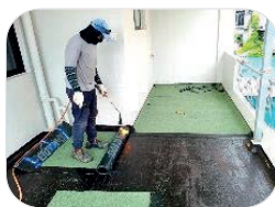
Torch-On Waterproof Membrane System
