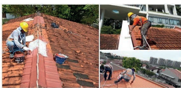
Pitched Roof- Water Leakage Repair
